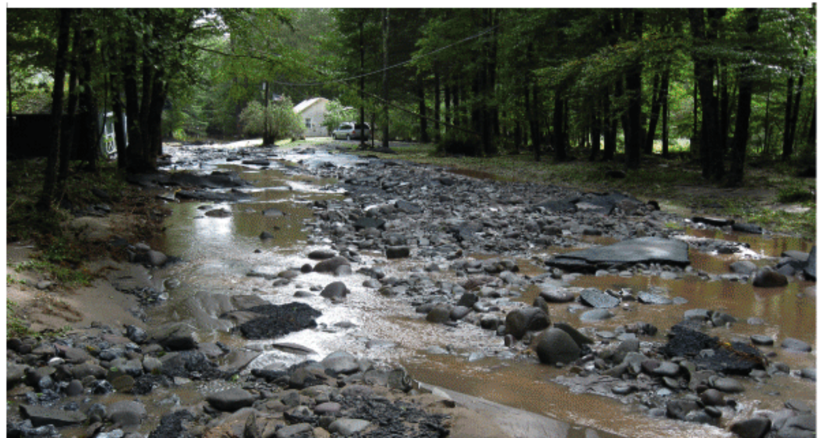
The same segment of Peekamoose Road that is pictured above, an hour after Hurricane Irene had hit the Catskills and the excessive water from the Rondout began to subside. Thanks to the dedication and efficiency of the Denning Highway Department road crew and the Town Board the road was temporarily repaired, and residents were able to travel through a few hours later.
