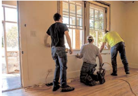
Workers installing new window
